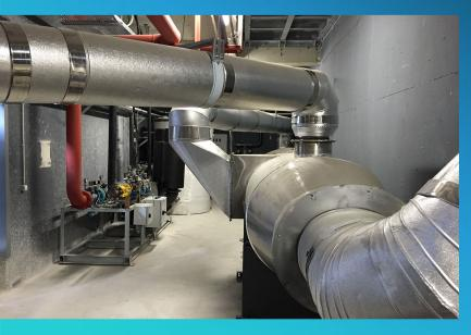
Drying of materials come from the surface cleaning process, before galvanizing in the kettle.
